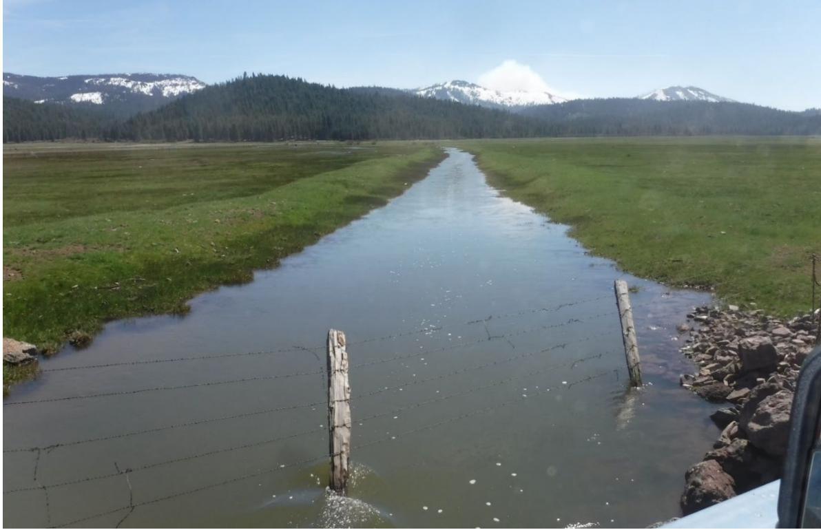
Photo 4: Active gully at Moonlight Road bridge, looking upstream. Note dredge spoil 'levees' to either side
