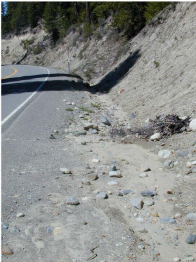
Eroding cutslope and inside ditch delivering water and sediment to a small stream channel.
