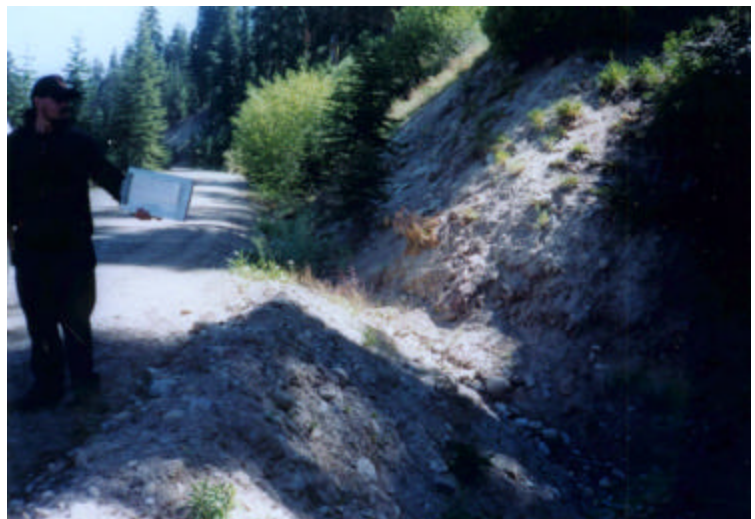
Inside ditch draining directly to a stream.
