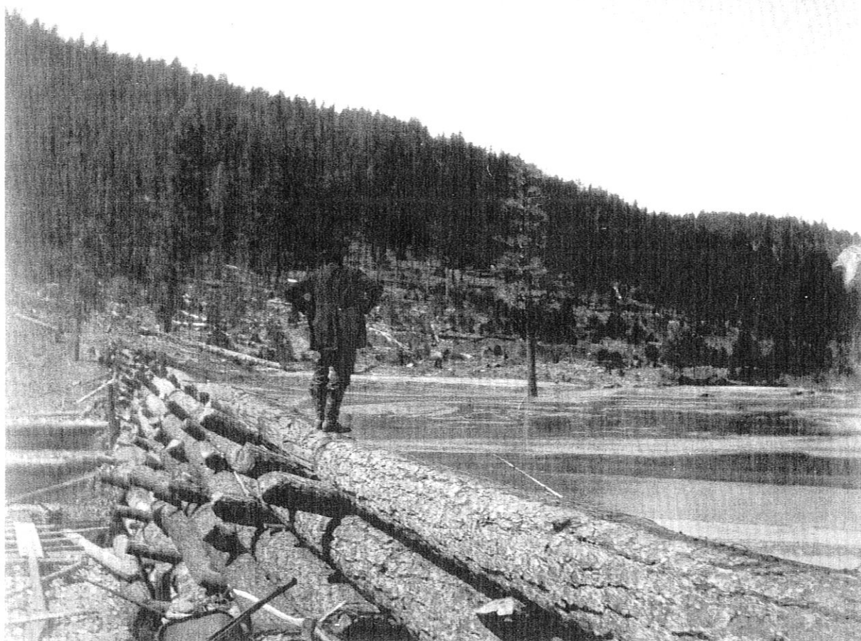
Figure 5. Sediment Deposit Behind Log Crib Dam at Green's Flat
