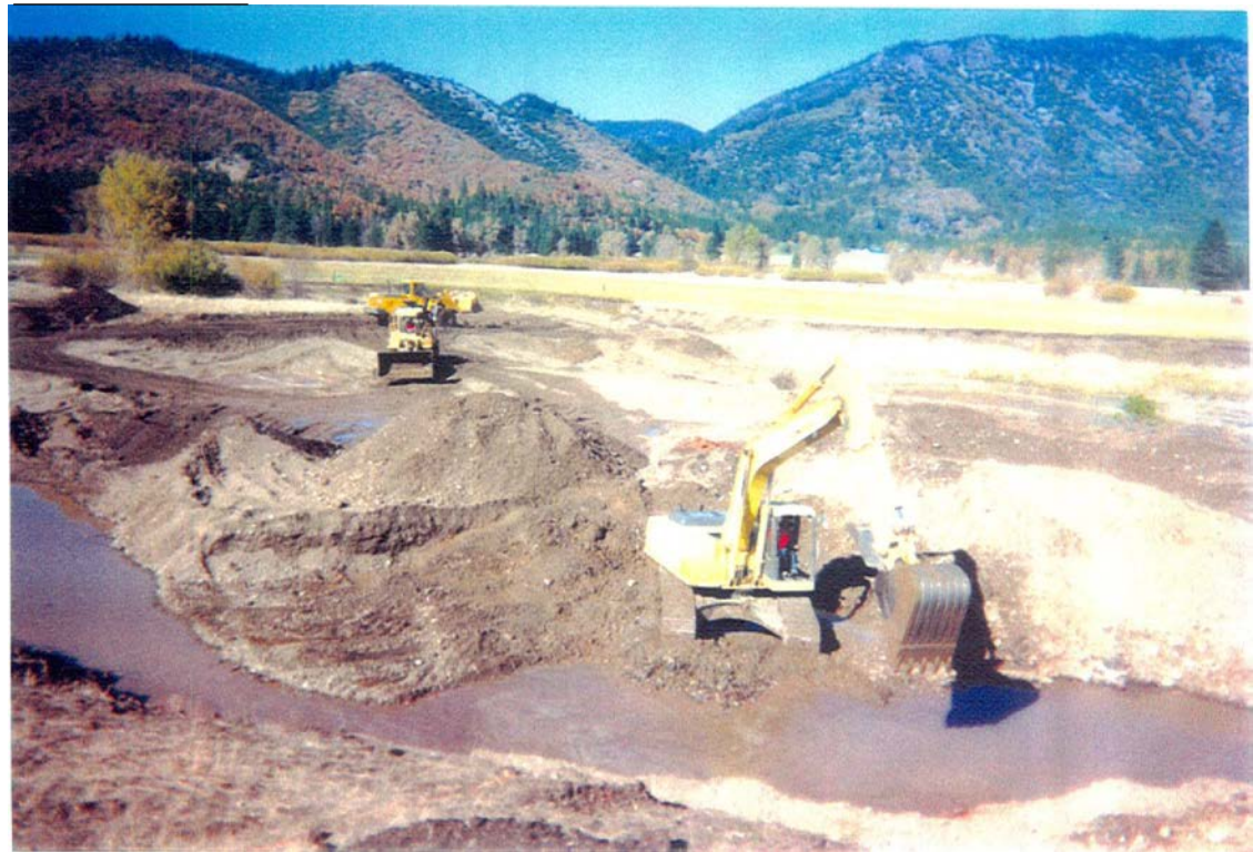
Fig. 3.14 Construction of the Ward Creek Project entailed excavating ponds within the gully (foreground), and using that material to build the gully plugs (background). Note that equipment haul routes are within the gully. While not shown in this photo, it should also be noted that Ward Creek is not flowing through the construction area — the new channel was constructed first.
