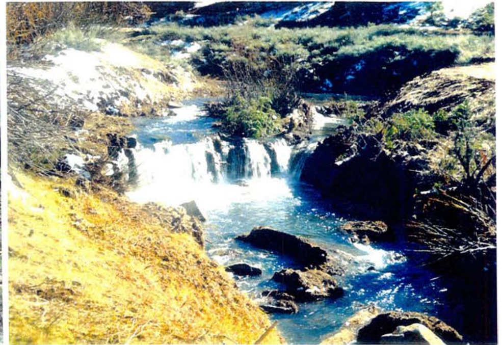
Fig. 1.5 Headcut treatment on Little Stony Creek, built in late 1996, was severely damaged during the 1997 flood.
