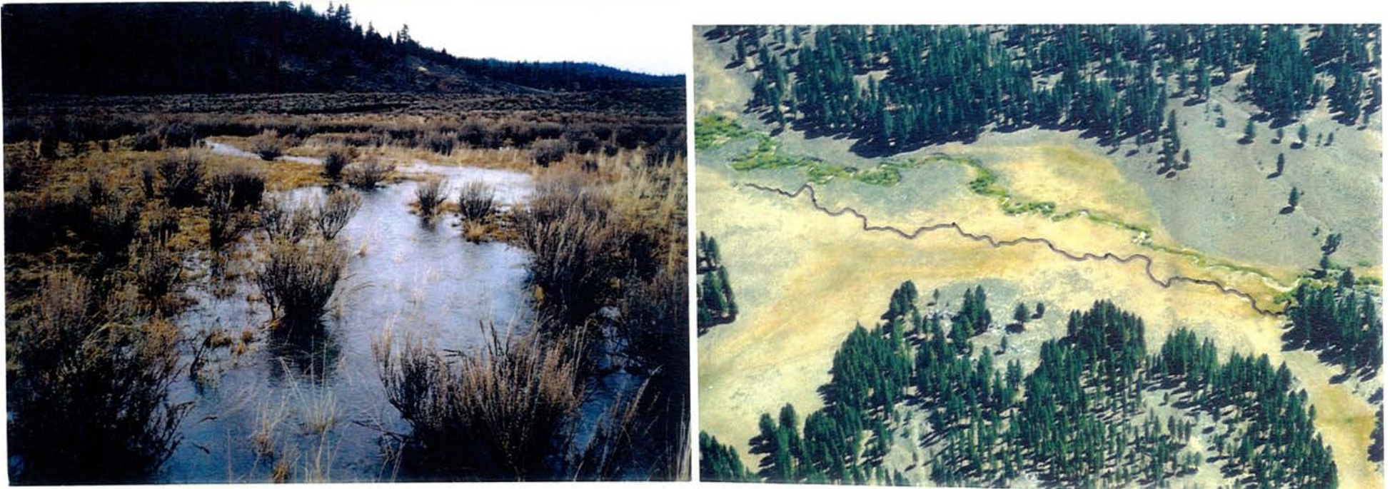
Fig.3.10 Using remnant channels. On the left, one year after construction, high water accesses the floodplain as it flows down a remnant channel used in the Bagley Creek project. On the right, in this pre-project photo, we've outlined the remnant channel to be used by Clarks Creek in conjunction with gully obliteration.
