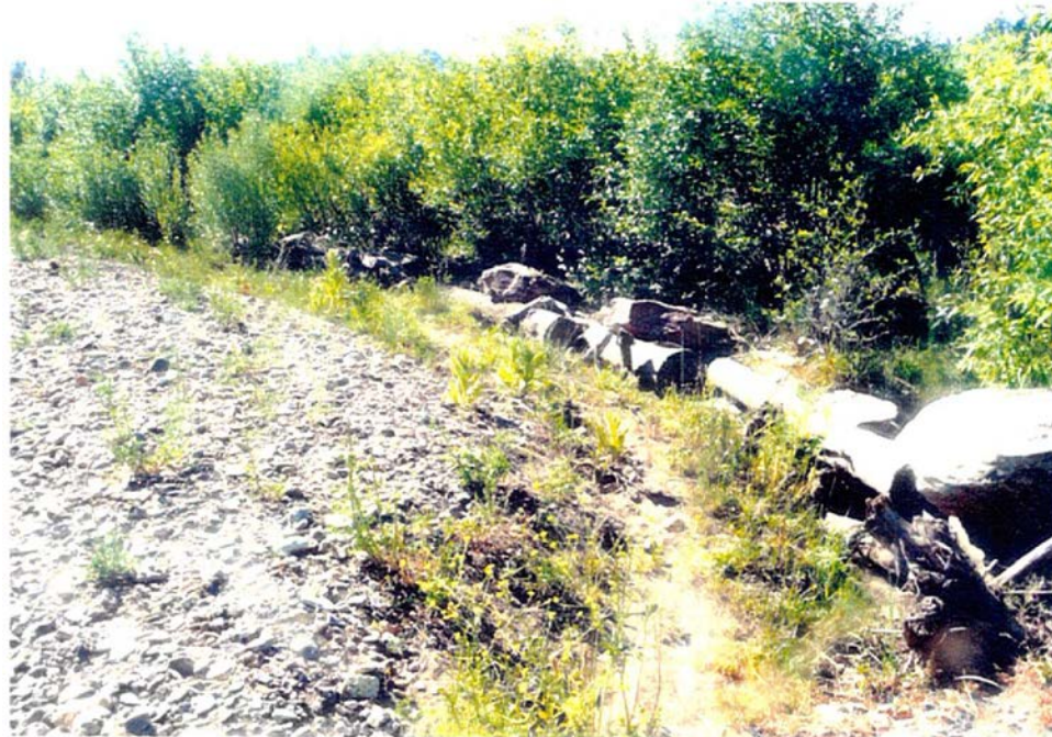
Fig. 2.2 This channel bank revetment structure was abandoned on Wolf Creek during the flood of 1995. Note the deposition of bedload.
