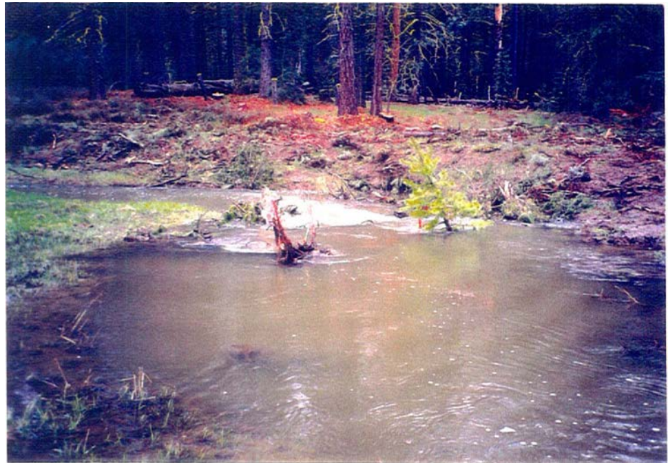
Fig. 3.20 (above) Debris jams were installed on Boulder Creek in 1997. The gully in this photo is six feet deep. Low flow water is not visible, but is flowing under and through the structure.
