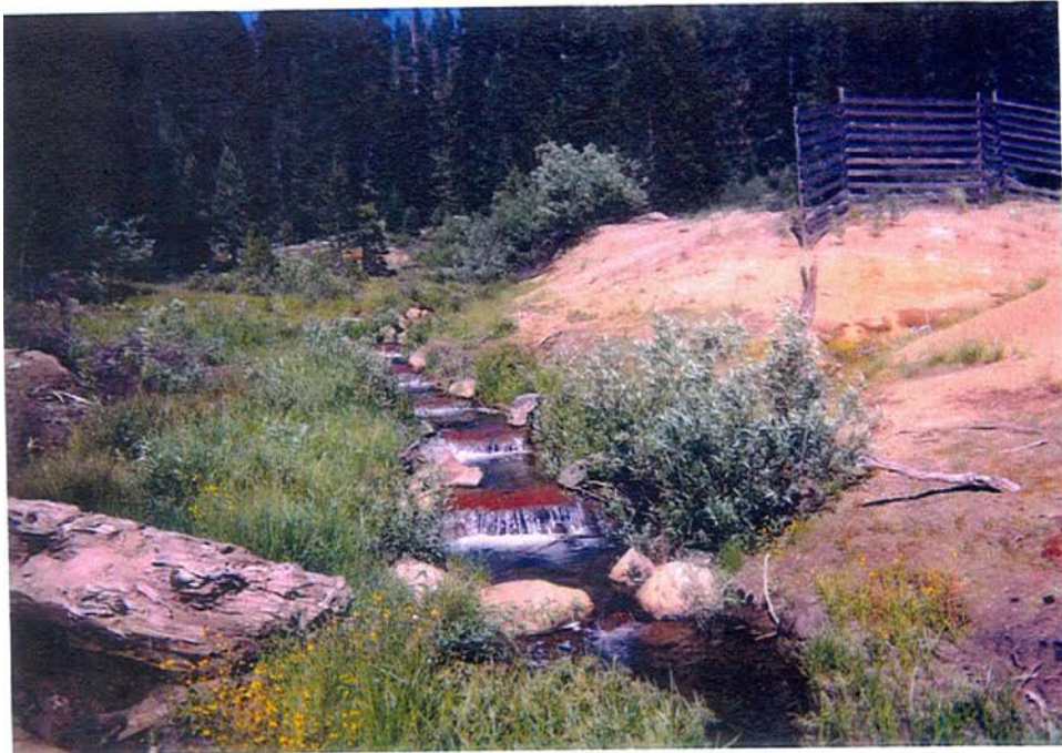
Fig. 4.4 A headcut step-pool treatment was constructed in 1994 on Dolly Creek as part of the Walker Mine Tailings Rehabilitation Project. The photo on the left was taken after the 1997 flood. Notice how the wide floodplain at the upstream end narrows down, thus directing flood flows through the steps and pools.
