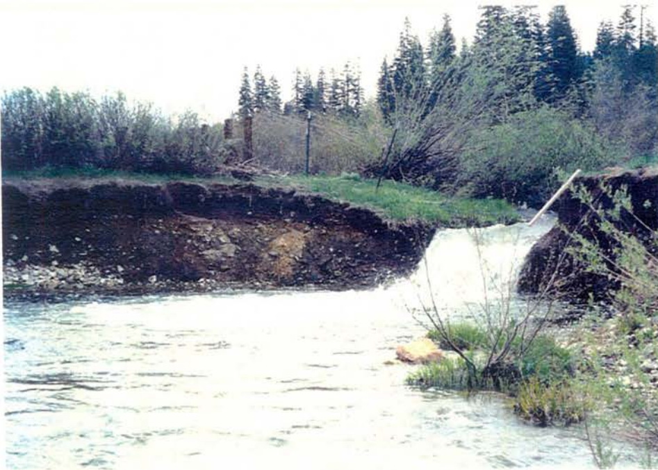
Fig. 1.4 This photo, taken in 1994, shows the headcut on Haskins Creek that threatened a wetland area. The CRM treated the headcut in 1994 using geomorphic technology. A flood in 1995 returned the repaired channel to its original condition.
