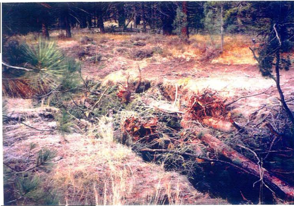
Fig. 3.20 (above) Debris jams were installed on Boulder Creek in 1997. The gully in this photo is six feet deep. Low flow water is not visible, but is flowing under and through the structure.
