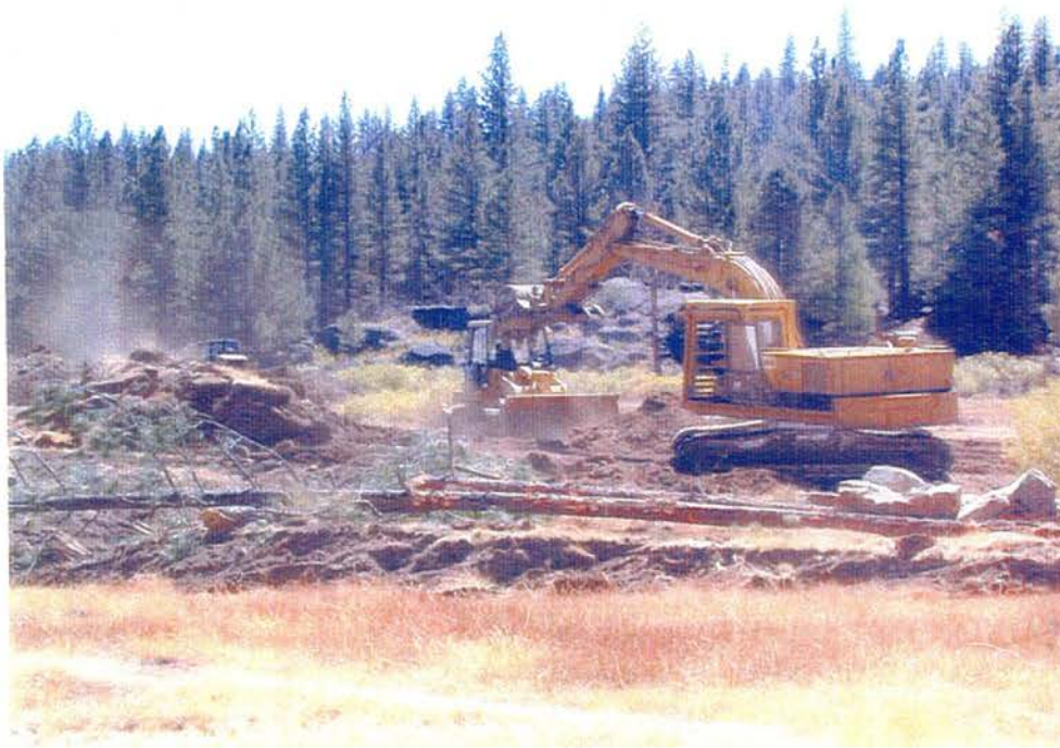
Fig.3.18 (left) This pile of sod and topsoil will be spread in the final stages of plug construction on the Clarks Creek project.
