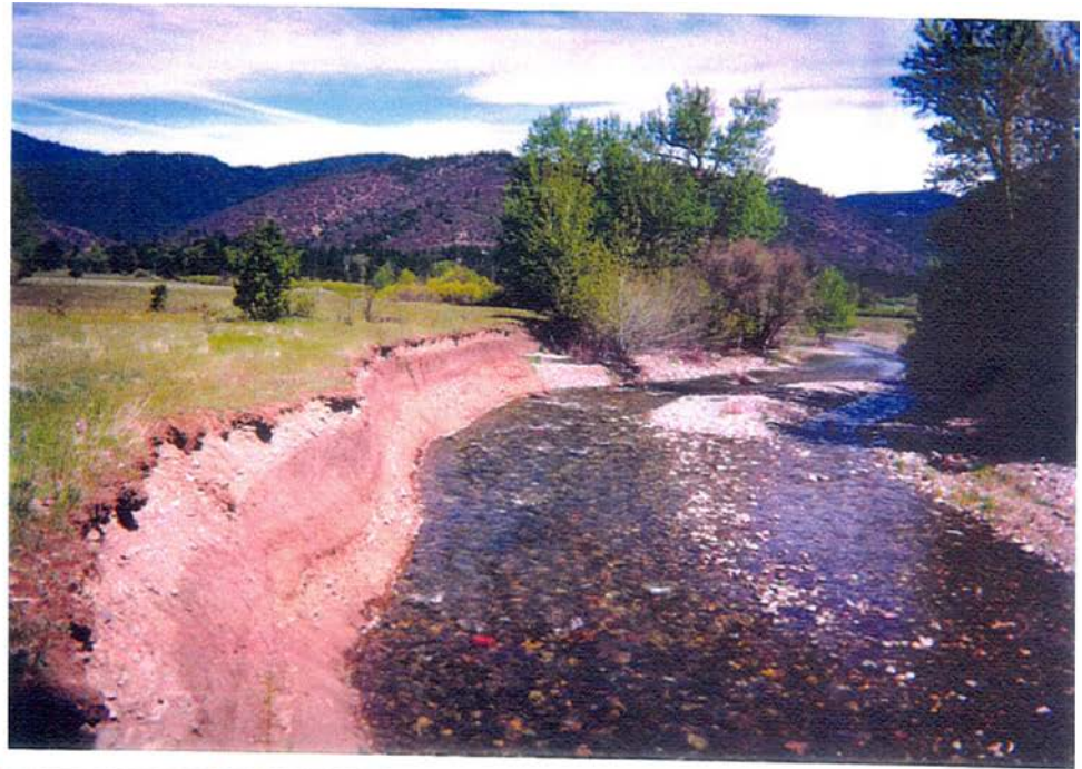
Fig. 3.15 These pre- (above) and post- (below) project pictures of Ward Creek are taken from almost the same vantage point (notice the cone shaped hilltop in the background). The post-project picture was taken in 1999, immediately after construction and shows how the gully has been eliminated by the plug. Since construction, the plugs are re-vegetating solely from large transplants and topsoil that was previously stripped from the construction site,
