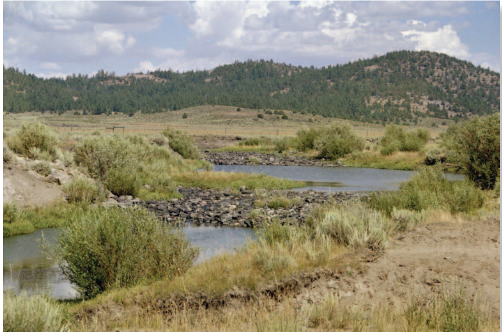
The middle two dams of the CRM's first project as seen in 2005. The CRM constructed four loose-rock check dams, replanted stream bank vegetation, and fenced the riparian corridor to keep livestock and vehicles out during a 10-year monitoring period after the work was completed. • Photo by Will Stockwin
