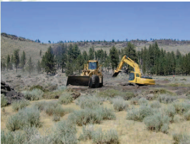
The project also required moving a section of county road 150 feet upslope, off the Matley's property and onto Forest Service land. The Plumas National Forest Beckwourth Ranger Station and Plumas County Department of Public Works led the road re-construction effort. Roadside revegetation was done by students from the Jim Beckwourth Continuation High School with locally collected seeds. • Photo courtesy of Feather River CRM
