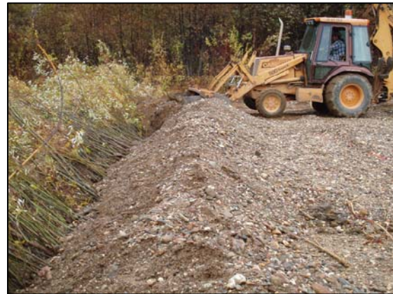
Packing down the soil in the willow trench
