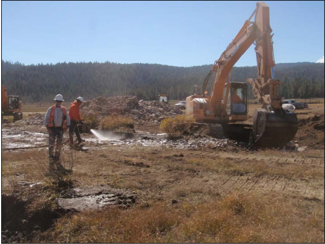
Construction of grade control structure on the Humbug Valley-Yellow Creek Restoration Project.
