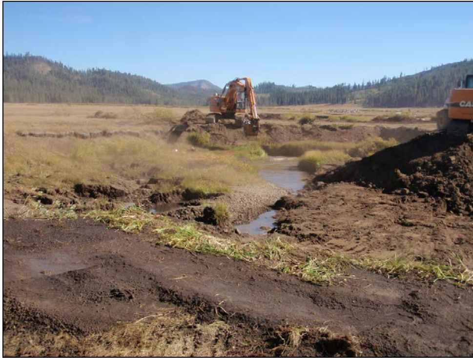
Pond and plug meadow restoration construction on Yellow Creek in Humbug Valley, Plumas County, CA. September 2013.
