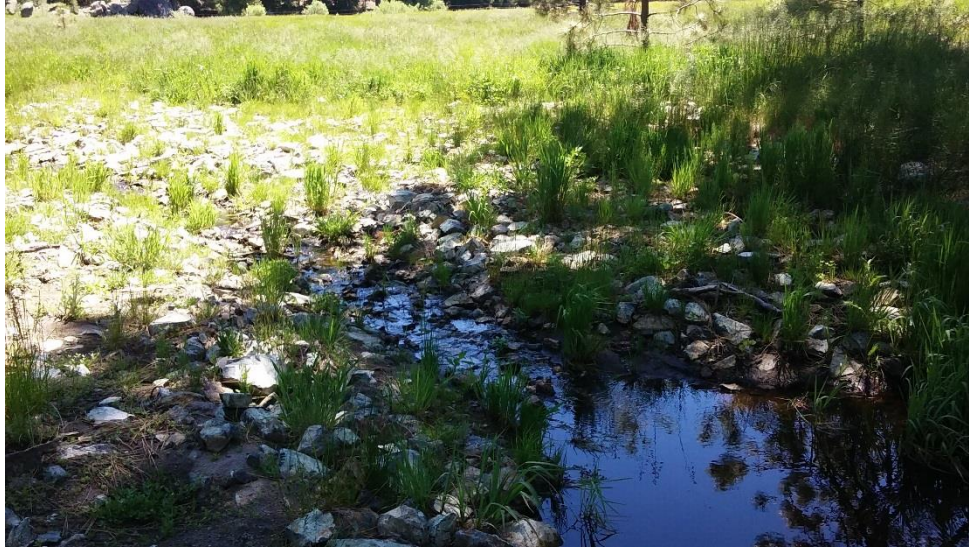
Figure 29. Detail of grade control looking upstream in July 2016. Native Carex has sprouted between rocks on the grade control structure. By July the stream is a series of small pools.
