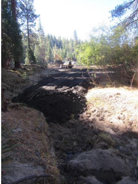
8b. Gully Filled, note location of large pine to the right
