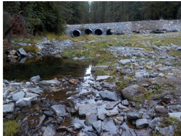
Photo 6b: Fish passable culverts, 2021 post-project
