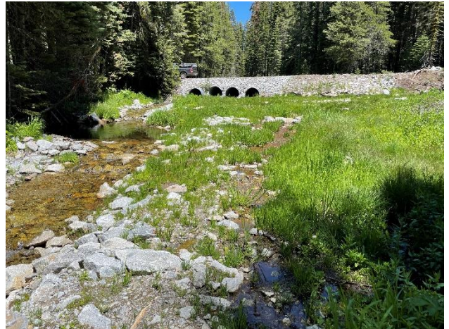
Photo 6c: Fish passable culverts, 2022 post-project
