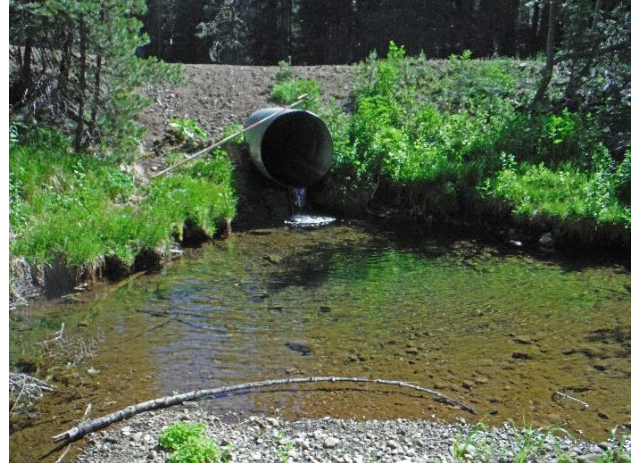
Photo 6a: Fish barrier culvert, 2020 pre-project
