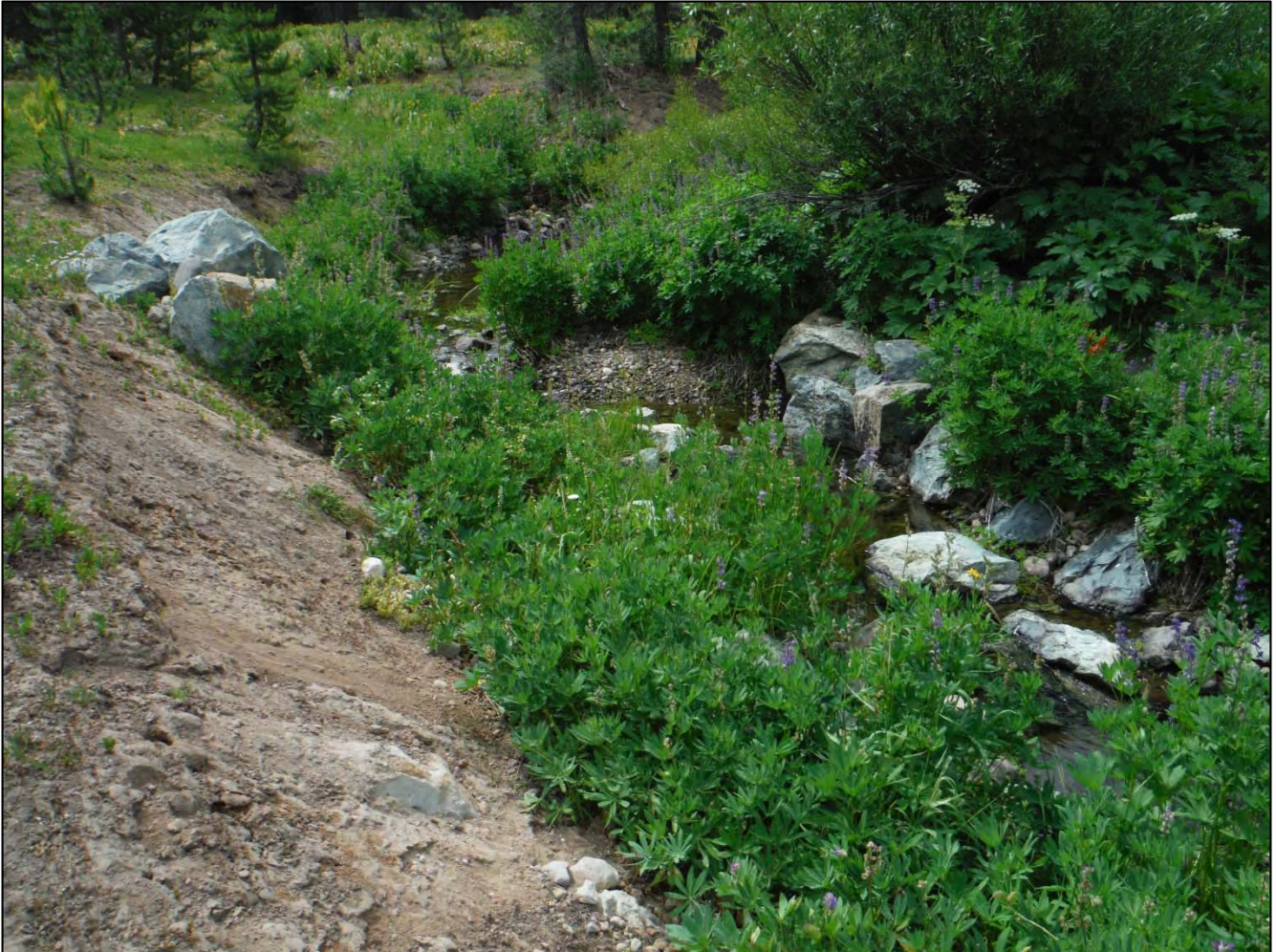
Photo #1: Middle Fork Cosumnes River gully in Foster Meadow near X-section #8. Breached rock check dam in photo center.
