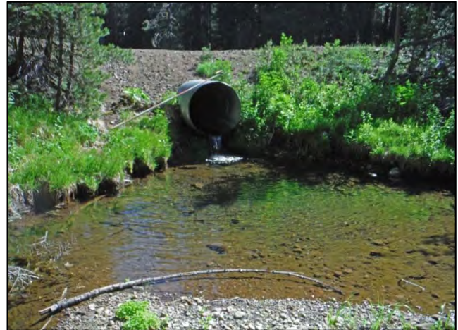
Photo #2b: FH 54 road crossing culvert outlet.
