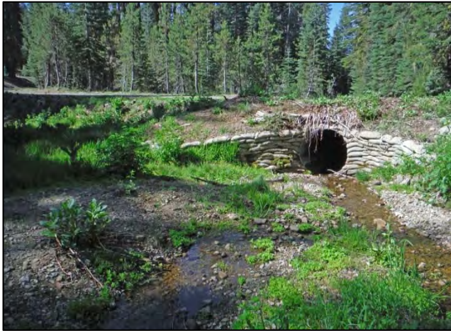
Photo #2a: FH 54 road crossing culvert inlet.
