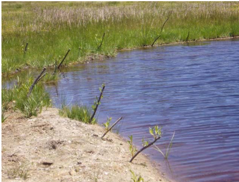
Photo 6. Edge of Pond in mid-meadow (Reach B2) showing growth of willow poles planted on the “plug” constructed downstream of the pond. Date of Photo- July 5, 2008.
